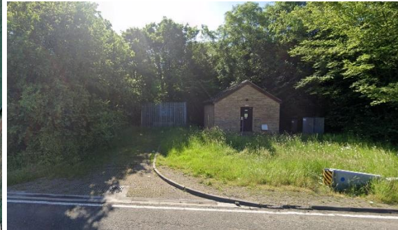
Figure 3-13 Photo of existing TS
